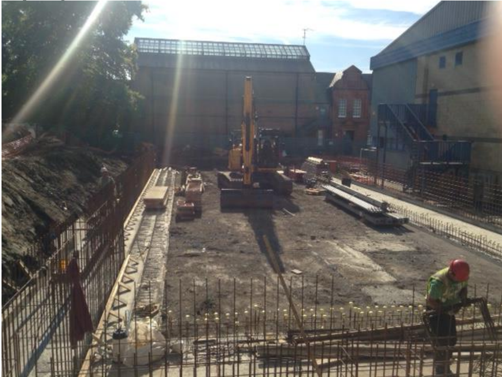
Preparing the site - late Autumn 2015
