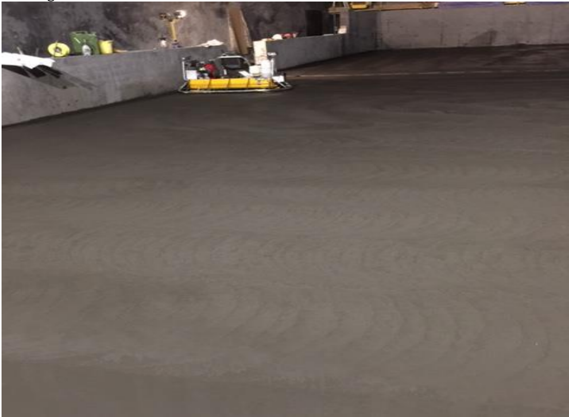
Pouring the concrete floor – Easter 2016
